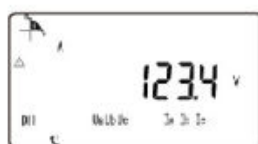
Voltage on A phase
